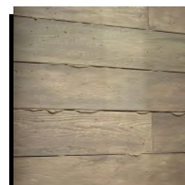
Board formed concrete
